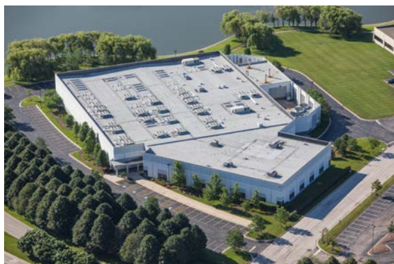
ByteGrid's Aurora, Illinois Data Center
